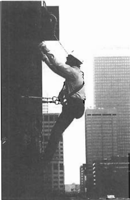
SRLs may be connected to a qualified anchorage or inserted to the back D-ring of a Rose full body harness.
